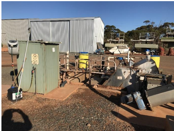
PLATE 31: Existing IDEA plant step screen arrangement (view to west). Isolate water and electrical services. Relocate bin to existing hardstand at completion of Works. Dispose all other equipment.
