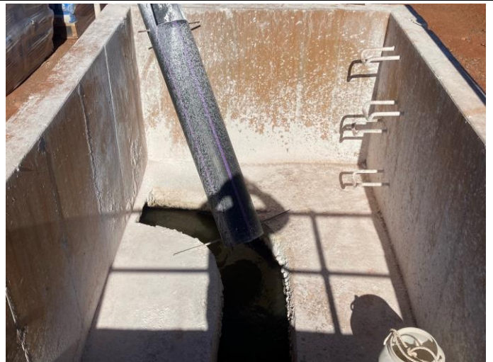
PLATE 4: Existing ponds access chamber. Manual lime dosing in place.
