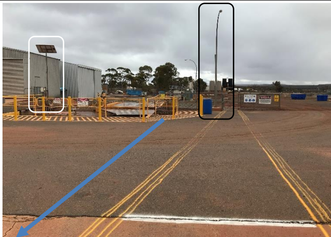
PLATE 15: Existing inlet structure (view top north). Light pole for relocation circled in black, instrumentation solar panel on pole to be decommissioned. Blue line for approx. DN600 sewer pipe alignment to existing liquid waste pit for removal and replacement DN600PE.
