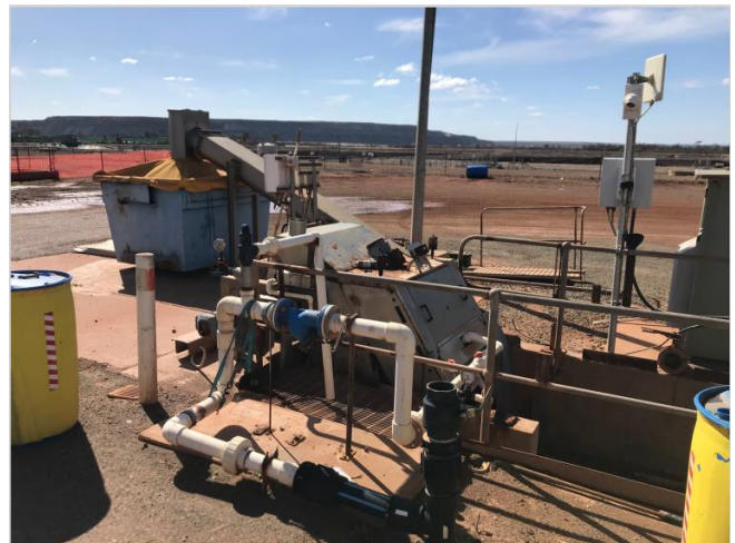
PLATE 32: Existing IDEA plant step screen arrangement (view to east).
