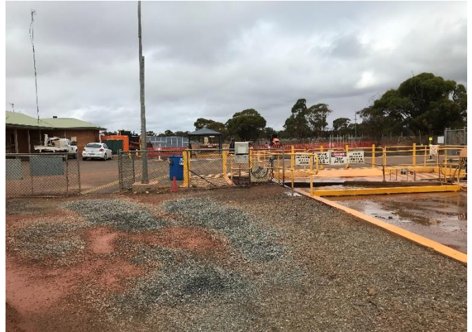
PLATE 20: East of existing hardstand. Light pole to be relocated, fence, bollards and guardrails to be disposed.
