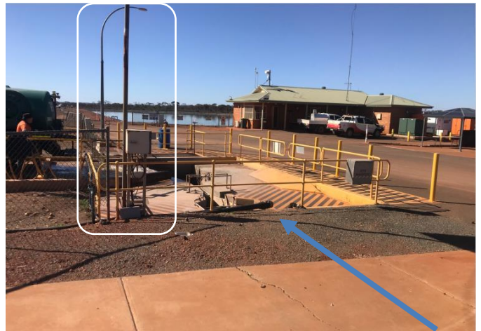
PLATE 10: Existing inlet structure (view to east). Operations building at right. Blue line for approx. DN750 sewer pipe alignment. Low fence, solar panel and equipment on left to be disposed.
