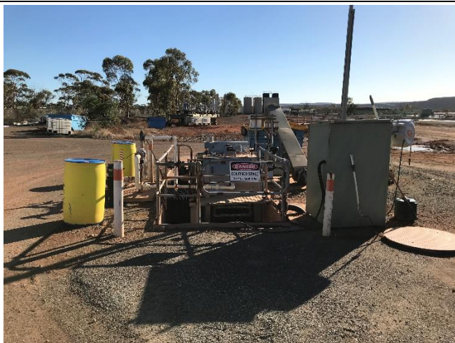
PLATE 33: Existing IDEA plant step screen arrangement (view to north).
