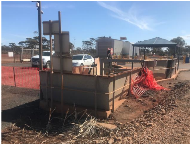
PLATE 38: Existing liquid waste discharge pit. All guard rails / barriers, signs and gate to be decommissioned and disposed.
