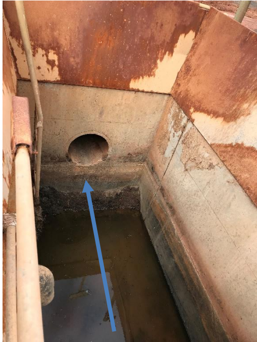
PLATE 39: Existing liquid waste discharge pit when isolated; pit currently has all sewer flows passing through – refer visible water mark. Desludge and dispose to WWTP sludge lagoons. DN600 AC pipe visible is connection point for new DN600 PE from new inlet structure. Break down concrete walls and backfill at completion of pipework.
