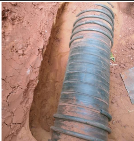
PLATE 11: Typical corrugated PE sewer pipe in Kalgoorlie; Existing DN750 assumed same. Pipe size and material to be verified on site.
