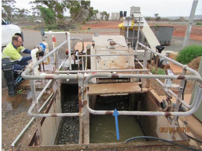
PLATE 35: Existing IDEA plant step screen arrangement internal. Decommission and dispose all equipment, guardrails, etc. Break through concrete pit to install DN600PE to existing and backfill.
