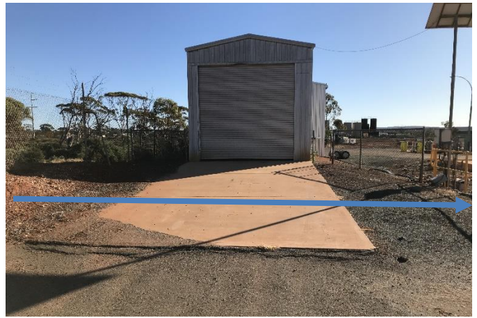
PLATE 8: Storage shed to north of entry gate (view to north). Concrete crossover to be protected or reinstated at completion. Blue line for approx. DN750 sewer pipe alignment. Low fence, solar panel and equipment on right to be disposed.
