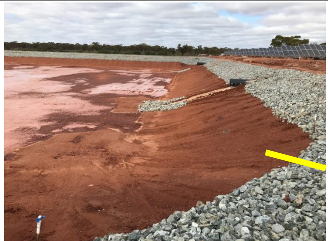
PLATE 24: Existing WWTP Pond 1A with clay lining and rock armour for overflow pipe inlet (shown as yellow line). Currently full of water.
