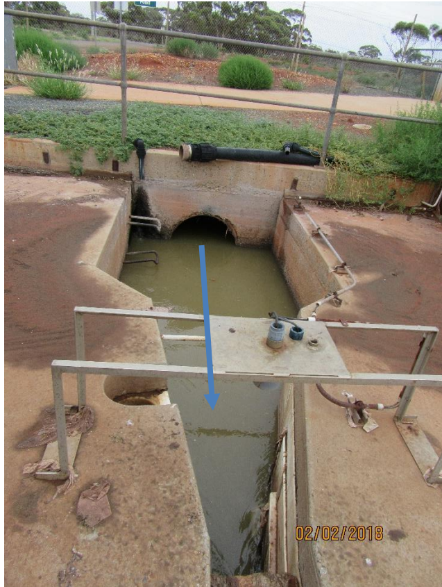
PLATE 25: Existing inlet structure concrete condition & casting layers visible (prior to yellow paint). DN750 inlet pipe at rear. Ultrasonic level sensor equipment and frame to be disposed, including cabling to solar panel and control cubicle on right (out of picture)
