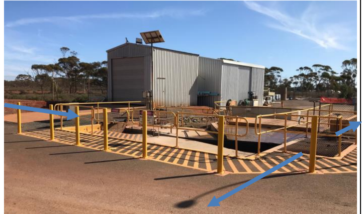
PLATE 14: Existing inlet structure, Blue line for approx. DN750 sewer pipe alignment and two (2) exiting DN600 outlets from the splitter chamber.
