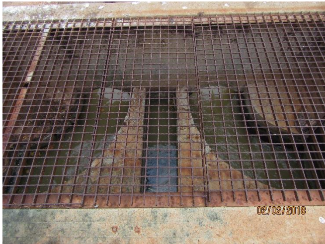
PLATE 29: Existing inlet splitter chamber – central pipe is decommissioned, right side (north) is isolated, left side (south) flows to ponds.
