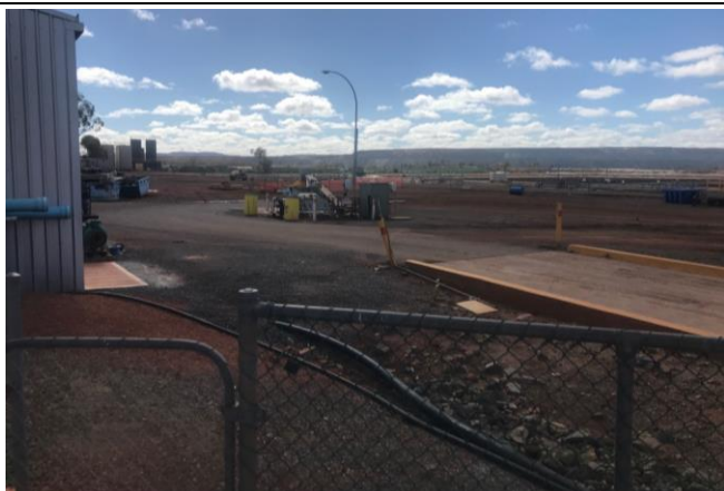
PLATE 17: View from shed crossover / entry gate to north. Existing truck hardstand on right to be retained for screenings bin. Existing IDEA step screen to the rear for decommissioning.
