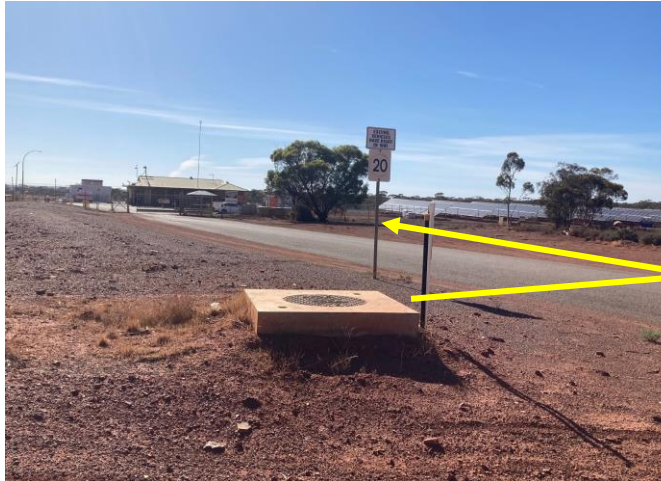
PLATE 1: Existing sewer access chamber T1 for Works isolation and temporary pump install. Yellow line for approx. location of temporary pipe route including sleeve under road (viewing east to WWTP). Liquid waste carriers and operators will be directed to gate on right (south) of temporary pipe.
