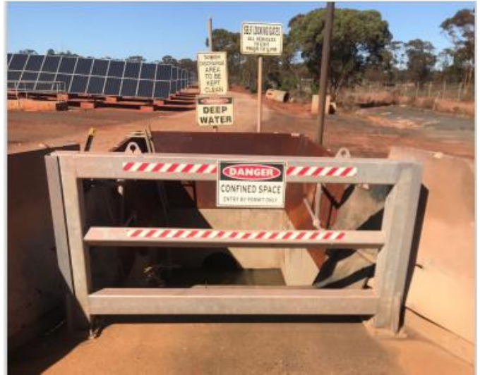
PLATE 36: Existing concrete liquid waste discharge pit. All guard barriers, signs and gate to be decommissioned and disposed.
