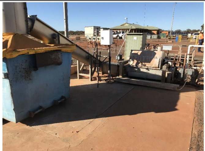
PLATE 34: Existing IDEA plant step screen arrangement (view to south).
