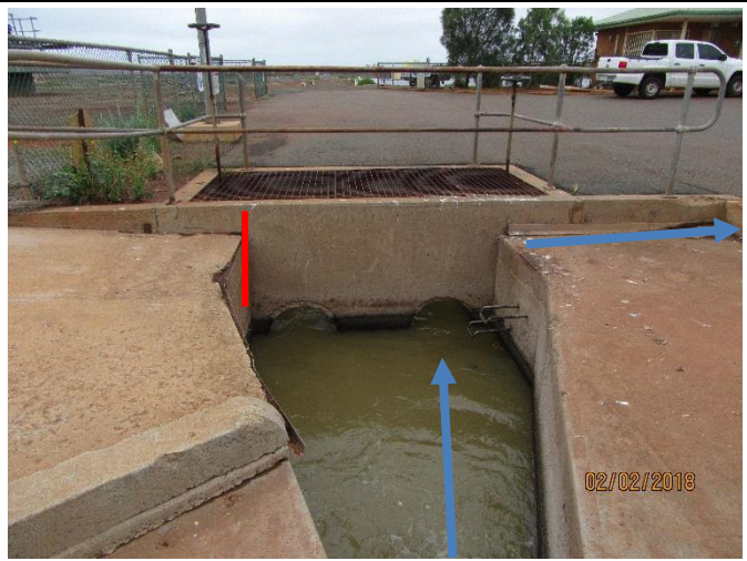
PLATE 28: Existing inlet has splitter chamber at end. Flow to north / left (IDEA plant) is isolated with manual penstock in the chamber. All flow currently directed south / right to ponds.
