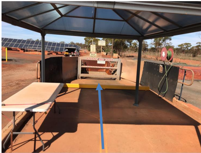
PLATE 37: Existing liquid waste discharge pit and apron. To be excavated for replacement of DN600 pipe.
